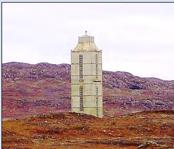
The deepest borehole ever drilled so far on Earth is the 12.3 km deep Kola Superdeep Borehole. This was drilled in the extreme north-west of Russia over more than 20 years, finishing in 1992. The borehole drilled around a third of the way through the continental crust, mostly through Precambrian granite and gneiss. One of the surprises was that the rock was still saturated with water deep in the borehole.
