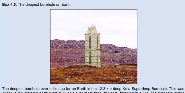
drilled in the extreme north-west of Russia over more than 20 years, finishing in 1992. The borehole drilled around a third of the way through the continental crust, mostly through Precambrian granite and gneiss. One of the surprises was that the rock was still saturated with water deep in the borehole.
